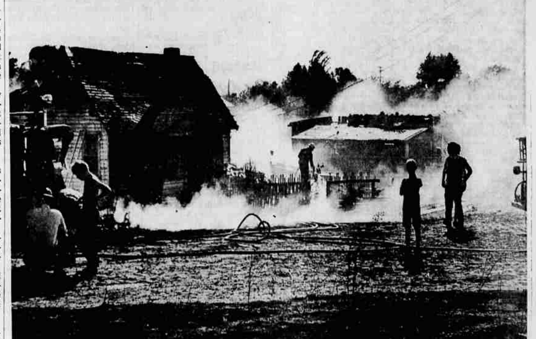
HOMES GUTTED—A fire destroyed one home and severely damaged another in a blaze which also burned 12 acres of grass yesterday. The homes, belonging to Elbert Garrison, 1487 1/2 Ridgeway st., and the other, belonging to Leftoy Fellows,
