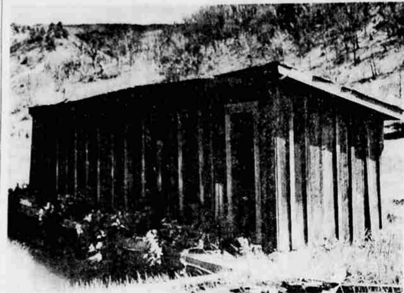
REMOTE BATH HOUSE—Near Klamath Hot Springs in northern Siskiyou county there still stands a small building used for changing into swimming suits for those who wished to swim in the warm pool. While the big bath house was farther up river, this small pool outdoors was a favored spot for many visitors. One visitor who frequented the small plunge was Amelia Earhart, who visited the spa many times before her tragic disappearance on an attempted round-the-world air tour with a pilot. The pair disappeared on the trip, never to be heard from again.
