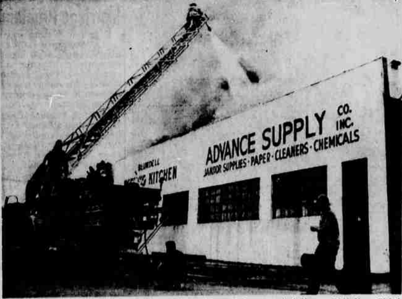
DESTROYED FIRM—Fire destroyed a janitorial supply firm and custom cannery in Salem, Ore., last Thursday. Estimated $100,000 damages were done to two businesses housed in same building. Battalion Chief John Settler fell 35 feet into flames but safely made his way out and sustained only minor cuts. (UPI)
