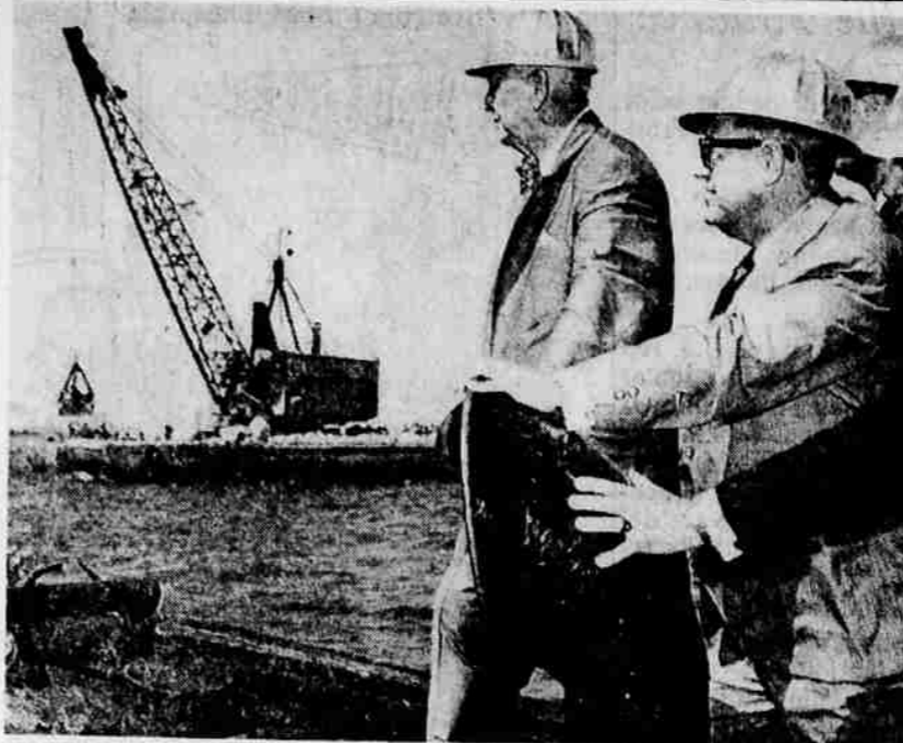
BUILDING FAIR SITE - Dan Kimball, left, board chairman of the California World's Fair, and Fred Hall, right, executive vice president and general manager of the fair, watch as the two-million ton of rock is placed on Pier J, site of the fair in 1967-68 at Long Beach, Calif. The 300-acre pier will be created mostly from actual ocean bed. (UPI)
