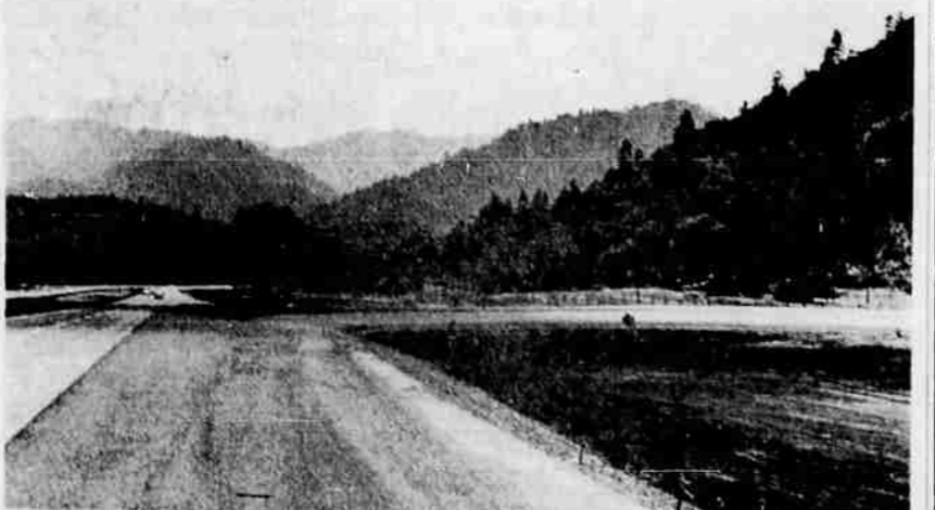
NEW FREEWAY INTERCHANGE — Motorists are now using the new Interstate 5 interchange at the Valley of the Rogue State park, although the on and off ramps haven't officially been opened yet. The ramps have been paved, but no signs have yet been erected. A State Highway department spokesman in Grants Pass said he thought a sign company strike was delaying the final stages of the project. He said no official opening date has been set but noted that motorists are free to use the interchange now. The above scene shows the off ramp for northbound traffic, which winds around under the freeway to reach the park on the south side. Prior to construction of this interchange, motorists had to get off at Rogue River or Gold Hill in order to reach the park.
