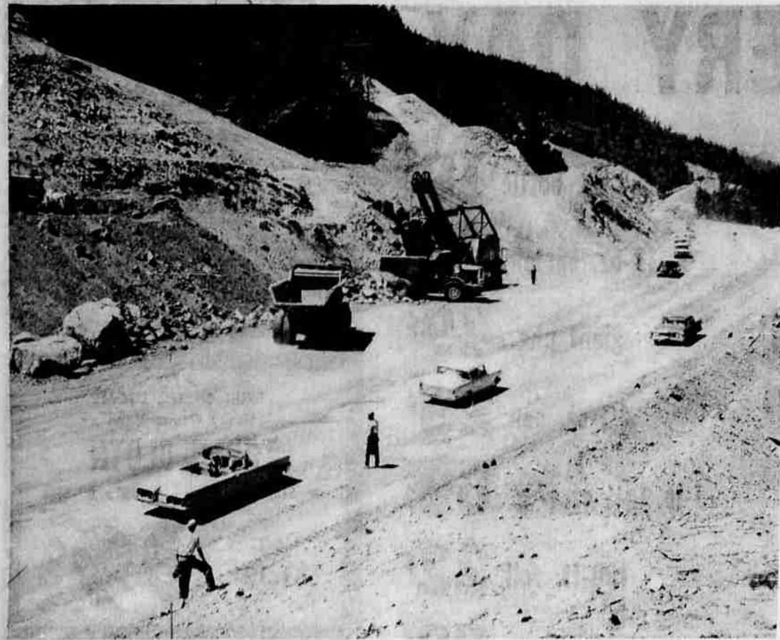
FREEWAY CONSTRUCTION - Work on Interstate 5 construction project south of Ashland interchange to Wall creek in the Siskiyou mountains is under way the entire 3.6 mile length. Clearing right of way is still being completed on the southern one-half mile. Peter Kiewit Sons' company crews, above, are removing material on the west side of Highway 99 at this point 1 1/2 miles south of Neil Creek. A shovel takes a five cubic yard bite to fill the dump trucks which transport the fill material across the highway. At left, one of the larger blasts sends up plumes of smoke and dirt as a rocky point is broken up. Smaller blasts are set off nearly every day, construction officials said. (Knackstedt photos)
