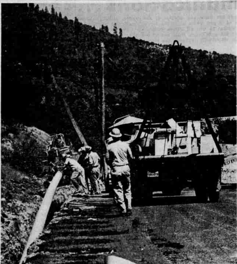
ENTER JACKSON COUNTY — Crews of gas line between Grants Pass and Medford, the Roy Price, Inc., company, Bakersfield, Calif., are shown as they installed a natural line in this picture taken Friday afternoon.
