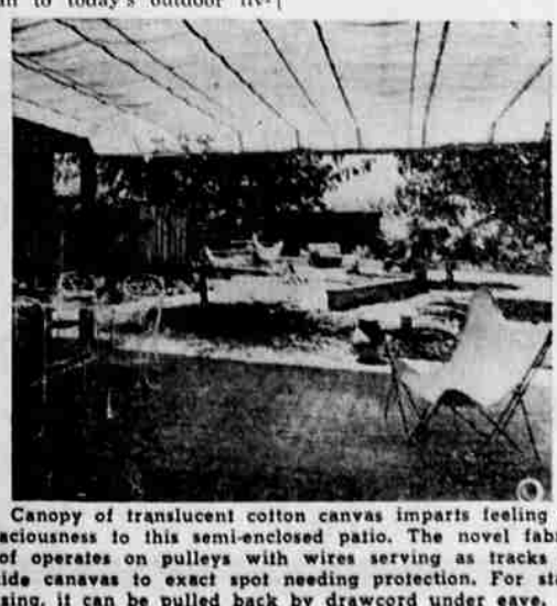
Canopy of translucent cotton canvas imparts feeling of spaciousness to this semi-enclosed patio. The novel fabric roof operates on pulleys with wires serving as tracks to guide canvas to exact spot needing protection. For stargazing, it can be pulled back by drawcord under eave.
