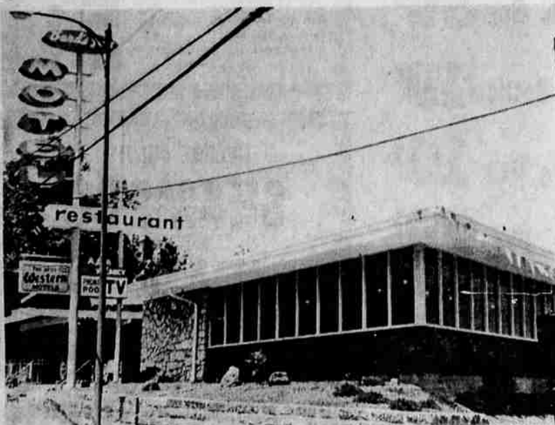
RESTAURANT NOW OPEN — The restaurant at the new Bard's Inn motel in Ashland opened last week. Both are located on the old Presbyterian church property at Helman and North Main sts. Cecil Halstead, formerly of Denny's in Medford, is owner of the restaurant, which is managed by Mrs. Pat Moultray. The main dining area accommodates 66, while an adjoining banquet room can seat up to 38.
