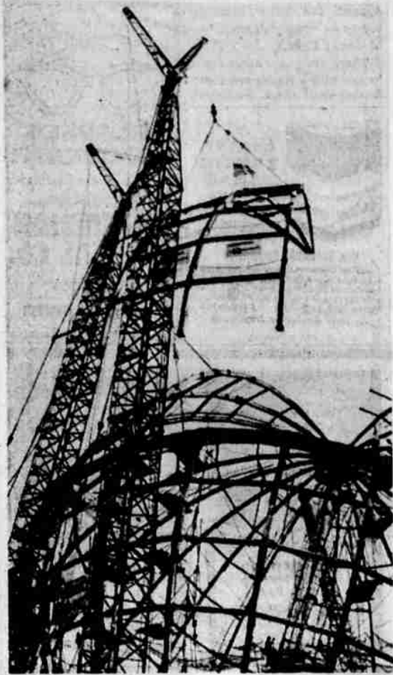
FAIR SYMBOL READIED —The last piece of the steel framework of Unisphere, the permanent symbol of the 1964-65 New York World's Fair, is swung into place at the fair's site in New York City. The 12-story structure is being built and presented to the Fair by U. S. Steel Corp. The final piece, representing the Pacific Ocean from 150 degrees west to 180 degrees (the international date line) and from the equator to the North Pole, carried the American flag as the last and highest piece of Unisphere. Construction of the framework took 110 days. (UPI)
