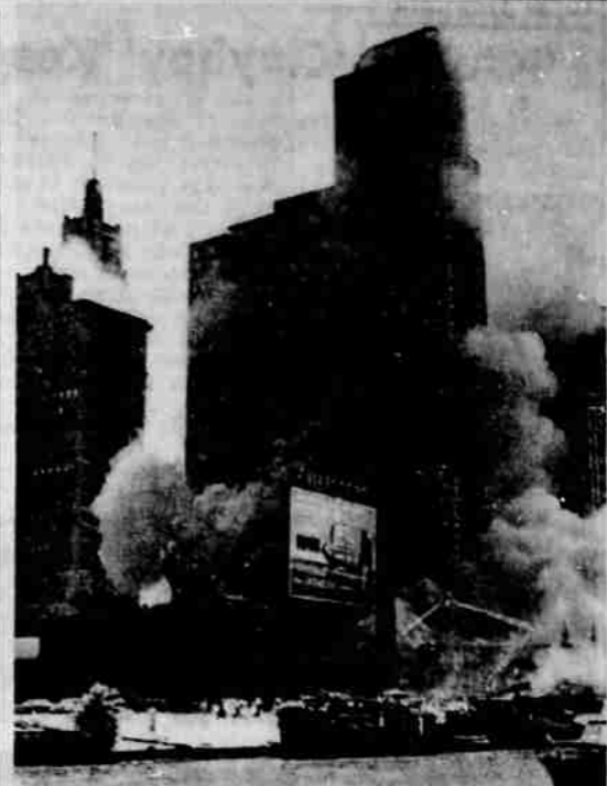
WAREHOUSE IN FLAMES —Billowing smoke encircles tall buildings as firemen battle a fire in warehouse on the south bank of the Chicago river in downtown Chicago. Fire boats and snorkel devices were called into action and firemen were able to confine the fire to the warehouse. Traffic on busy Michigan ave. was suspended due to the heavy smoke which settled over the city. (UPI)
