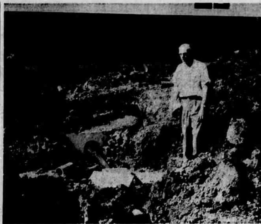
INSPECTING SYSTEM —Orie Moore, senior sanitarian with the Jackson county health department, looks over a private septic system being installed at a rural area home. The septic tank may be seen partially covered by earth near the center of the picture. The smaller container in the foreground is the distribution box.
