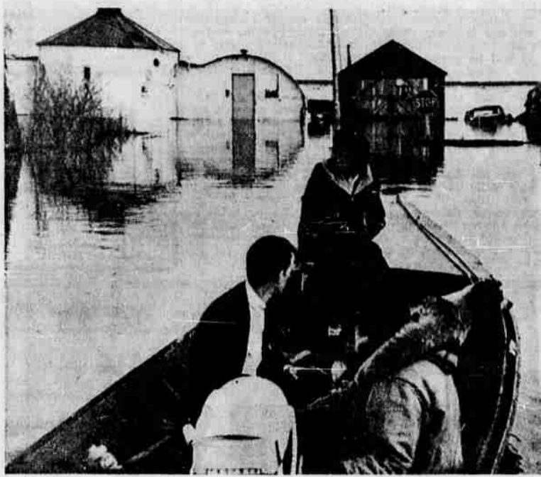
TOWN INUNDATED —The worst flood in 18 years leaves about five feet of dirty water over Bethel, Alaska. Residents are shown above using boats to survey the damage. The flooding in the small town on the western tip of Alaska is caused by massive ice jams 10 miles down the Kuskokwim river. Navy planes are trying to shake the ice loose by dropping bombs on the jams. (UPI)
