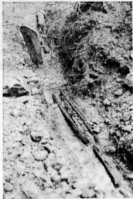
This photo shows the mine's old raceway with riffles as unearthed by Reynolds, who may be seen working in the background. Reynolds found the old mine when he spotted some rotting timbers sticking out of the bank along Briggs creek.
