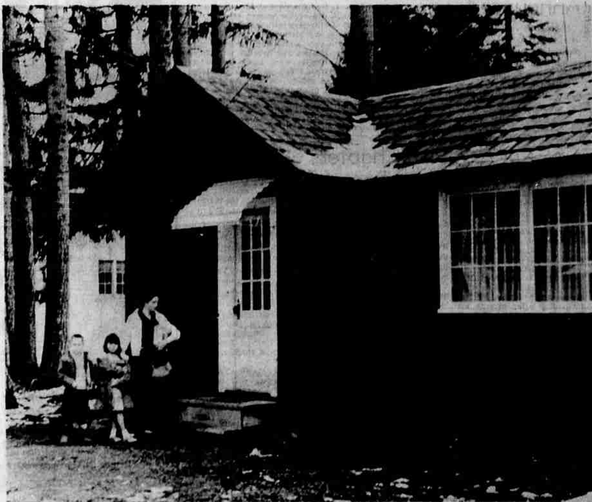
The Prospect branch library building was constructed by the residents of the community as a volunteer effort. The building was started about three years ago, and a wing added last year. In most instances, towns of the outlying areas in Jackson county supply quarters, and the main library provides the books and a branch librarian. Open house for the Prospect library will be held Tuesday, April 23, from 12 noon until 4 p.m.
