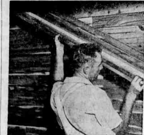
AROMATIC CEDAR — New, fragrant closets from old! This aromatic red cedar closet-lining can be installed right over old walls and doors. The handsome lining helps protect valuable clothing from moth damage and keeps them fresh and gently-fragrant.
