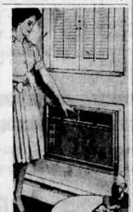
SOLUTION —Built in comfort: a through-the-wall installation of a room air conditioner may prove to be a permanent solution to the problem of year round comfort. Built-in units do not block the window and fit nearly-flush with the wall.
