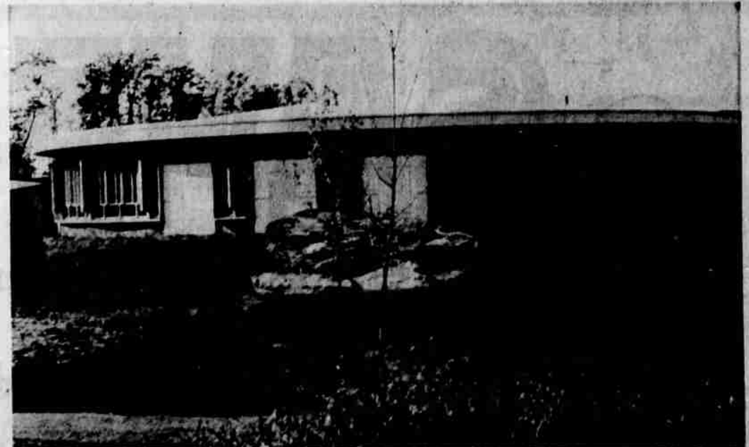
The library is more and more becoming an important part of any high school, and in many cases is now in a central location. This is the library building at the Newton High school in Newton, Mass. Surrounding the library are other buildings housing various departments. Pictures were taken by James L. Payne, Salem, architect, who accompanied educators on the trip.
