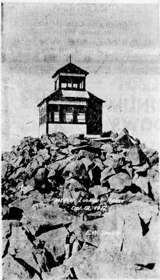
This is the lookout house constructed on Mt. Pitt in 1917. The guy wires had been attached and secured against the storm when this photo was taken Oct. 12.
