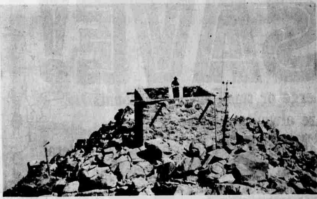
This photo shows the stone foundation constructed for the second lookout house which was built on Mt. Pitt in 1930. Smith also worked on this project, abandoned many years ago.
