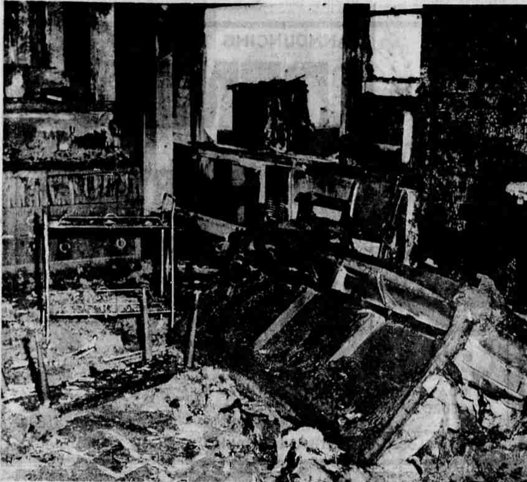
CHARRED INTERIOR - Fire, which started up again after it was thought to be extinguished, caused extensive damage to the penthouse over the Wilson-McCabe Refrigerating company early Saturday morning. Sawdust
