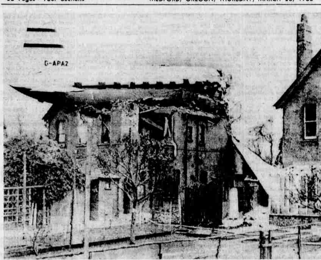
ROUGH LANDING - Wreckage of a Varsity training plane perches atop this suburban house in Gloucester, England, after a crash which killed test pilot Russell Palmer and assistant test pilot C. Thomas. Families living in the house miraculously escaped death. (UPI)
