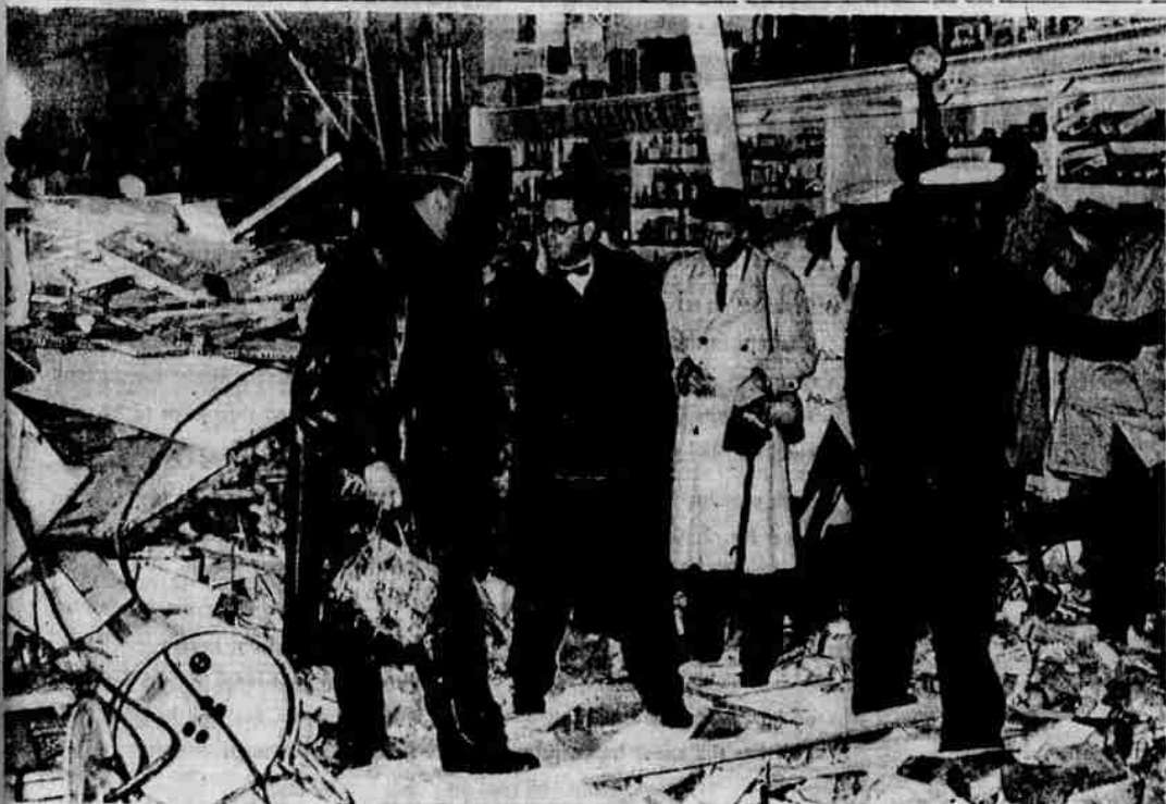
DEBRIS OF DRUG STORE - Mayor Robert Welch (second from left) talks with policemen who had been gathering up women's purses from debris of drug store in San Jose, Calif., Saturday after a boiler exploded in the basement of the building, killing three persons and injuring some 72 others. The building was shared with the J. C. Penney's store and both establishments were crowded with shoppers when the blast occurred. (UPI)
