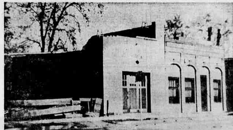
PARTIALLY DEMOLISHED — The old Yreka fire hall is shown here as demolition work was in progress recently and the second story had been removed. The adjoining building on the right was once a furniture store, but more recently was used as a residence.
