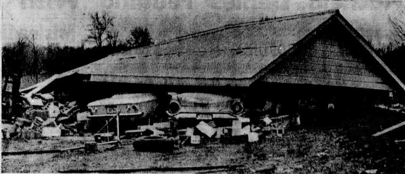
TORNADO DAMAGE—Tornadoes which hit Mississippi, Alabama and Tennessee Monday were blamed for four deaths and more than 20 injuries as the threat of more twisters hung over the Southland. Above, a garage is shown collapsed on two cars at Cedar Grove, Tenn. (UPI)
