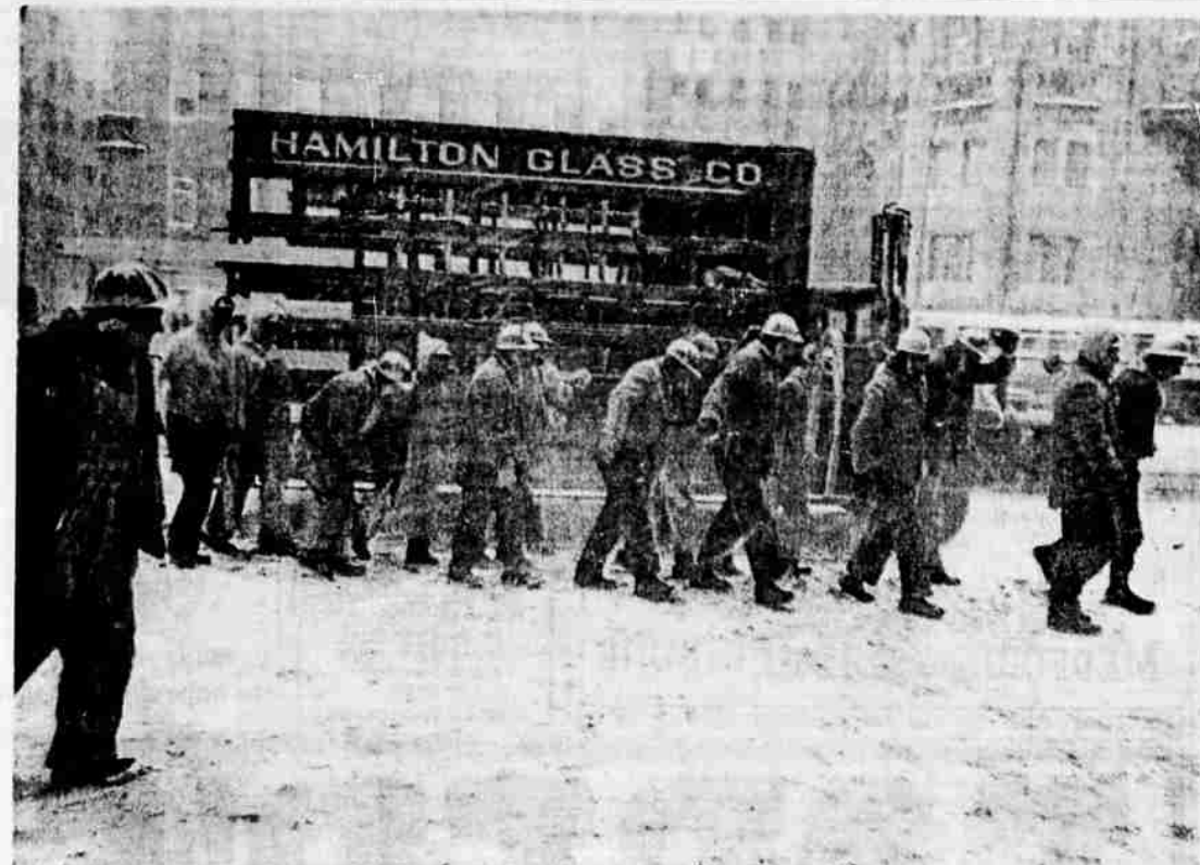
GLAZIERS CARRY GLASS - Looking much like a drill-master watching his section march through snow in neat columns of two, a foreman directs fourteen glaziers as they carry a 700-pound pane of glass to a building under
