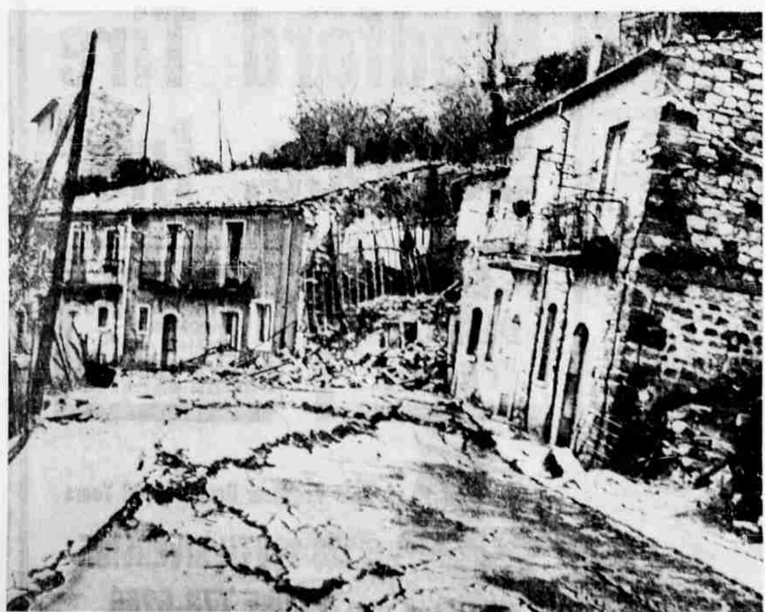
POPULATION EVACUATED —Cracked roads and collapsing houses due to landslides in the town of Caposele near Naples are shown in this picture taken late last week. The entire population of the town, as well as others in southern Italy, had to be evacuated. The landslides came after torrential rains which climaxed a cold wave. (UPI)
