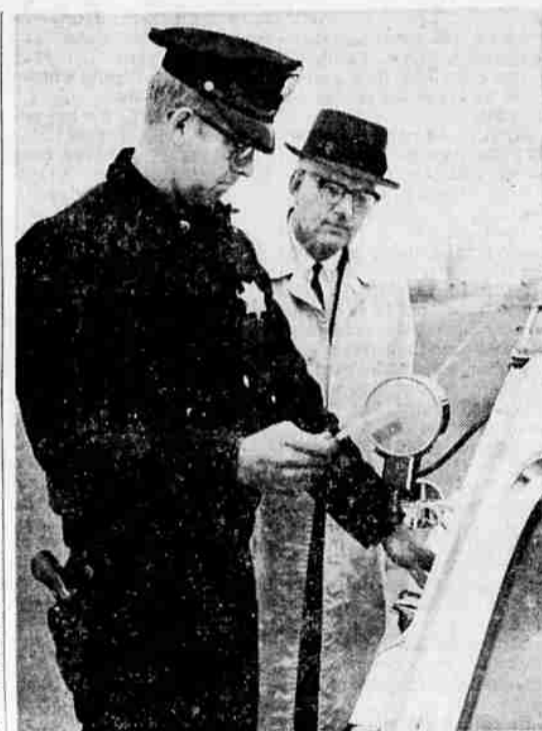
HOLDS TUNING FORK —As Police Chief Charles P. Champlin looks on, Officer Jerry Butler holds the tuning fork in front of the radar unit's transmitter-receiver to see that the instrument is operating accurately. When the receiver picks up the fork's particular vibrations, they are registered at a certain speed on the radar meter, which is kept in the front of the patrol car. (Knackstedt photo)
