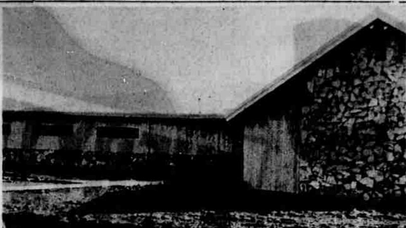
NEW CHURCH—The Church of the Nazarene, Evergreen lane, Yreka, is in its new building valued at $72,000. The structure include 14 classrooms and a sanctuary which seats 200. The church has both a grand piano and electric organ. Pews are now being constructed by the congregation members. The new building is of wood, concrete and rock.
