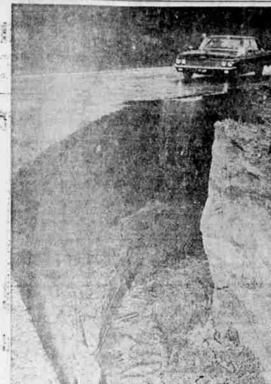
ROAD'S END - Warm rains have washed away this section of a street in a residential area in Salt Lake City, Utah. A police car is shown guarding the gaping hole. (UPI)
