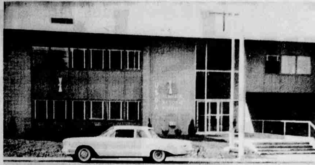
NEW YREKA BUILDING—This is the new home of the Klamath National forest offices. The building is on Highway 99 South in Yreka. The building was constructed by the Garnet Construction company of Sacramento under the General Service Administration of the Wells Fargo bank. It is leased to the forest service for a 10-year period with an option of further leasing. The personnel number 100. They moved into their new quarters in January and held open house on Feb. 2.
