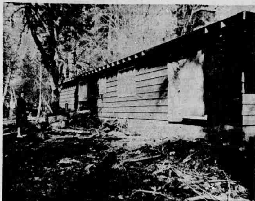
DEBRIS NEAR HOUSE —An Eagle Point area resident points to concrete steps which were washed away from the door, now boarded up at the front of the house. The steps were lodged against a tree. The house had been lived in about three weeks before the Dec. flood, and a once landscaped yard became littered with debris from Little Butte creek.
