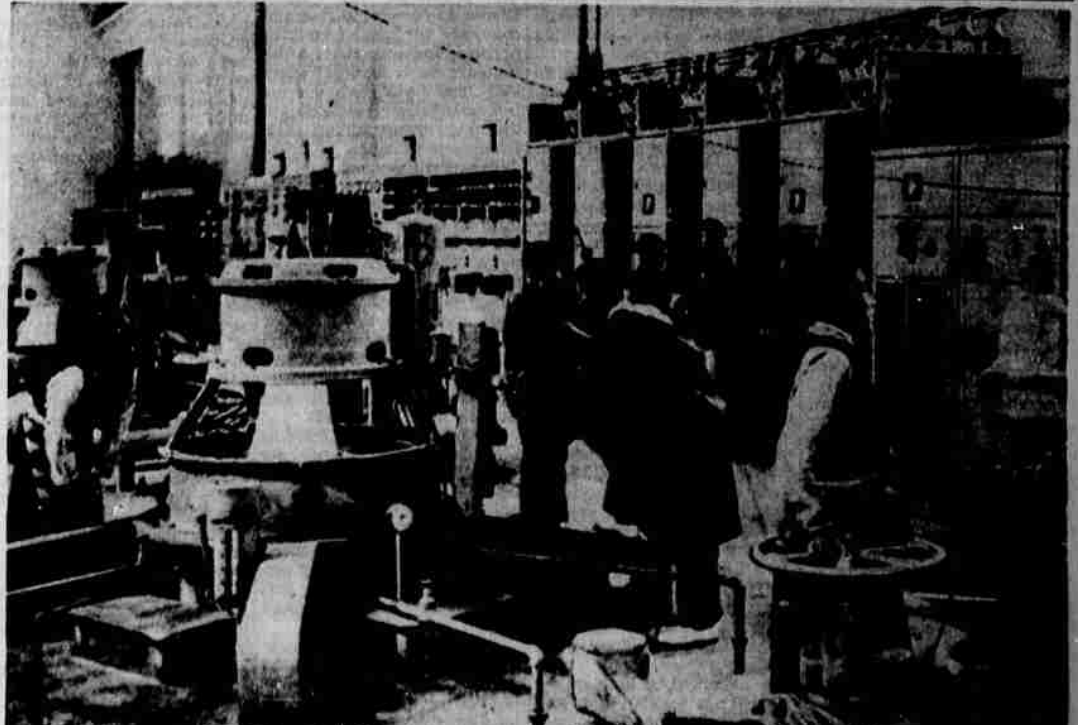
The Ngajim hydro-electric power station in Lhasa, Tibet, is a sign of the iron hand of progress in Communist-ruled Tibet. This picture, from an official Communist source was taken prior to October, 1961. (UPI)
