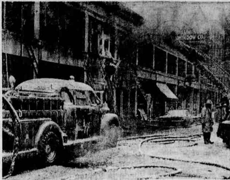
BATTLE FOUR-ALARM BLAZE —Firemen battled a four-alarm blaze in downtown Minneapolis early Saturday in near blizzard conditions. The temperature hovered around one degree above zero and fine powder snow was driven by 20-25 mph winds. The origin of the fire in the most packing center of town has not been determined.—(UPI)
