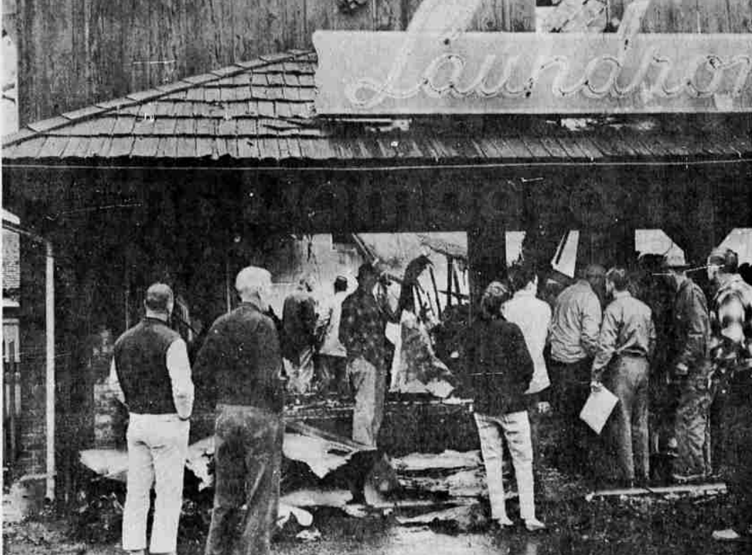
BUSINESSES DAMAGED —Four firms in one building across from the Big Y Shopping center, were destroyed by fire early Sunday morning. Burned in addition to the Big Y Laundromat (shown here), were the Frank Boone Barber Shop, Virginia's Big Y Beauty Salon, and the Big Y Cleaners. Firemen saved some of the equipment in the barber and beauty shops and falling debris damages some of the equipment in the laundry. Cause of the fire has not been determined. (See pictures on page 2.) Knackstedt photo
