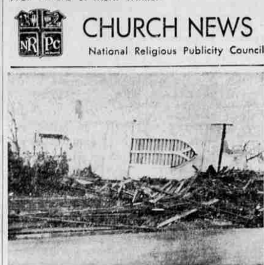
OLD CHURCH—All that remained of the former building of the First Presbyterian church in Ashland this week was the old bell tower, which is shown lying on its side. The church was a landmark in Ashland for a number of years. The property was sold to make way for a new motel.
