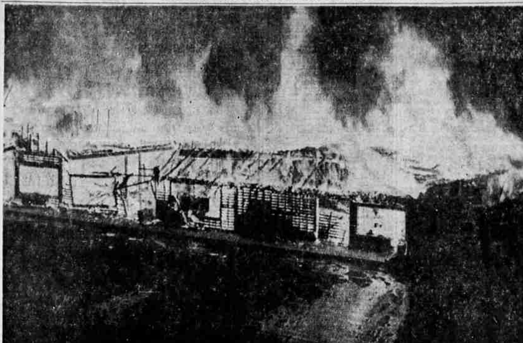
STRUCTURE DESTROYED —Damage estimates ranged as high as $400,000 from a fire which destroyed the Pines Shopping Center at Bass Lake, Calif., Tuesday night. The
