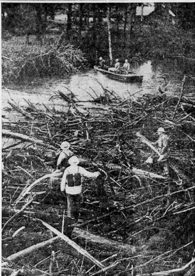
STREAM CLEANED — A corps of Engineers river launch assists Oregon state highway department workers to clear a log jam on the Tualatin river at Tualatin. The piled-up debris threatens a bridge and has already broken four pilings on the wooden span. Logs are from timber blown down in the Oct. 12 storm. (UPI)
