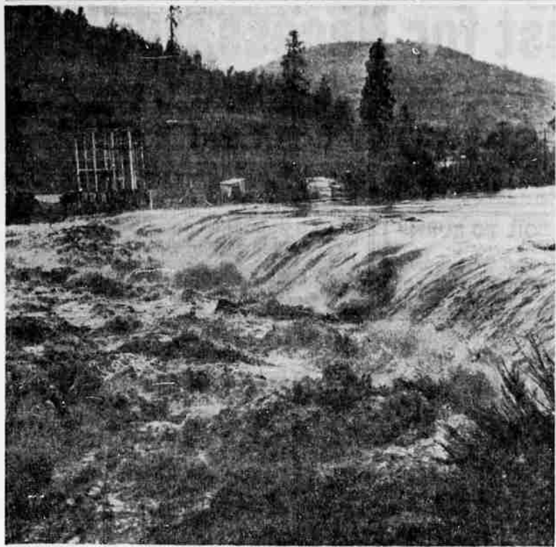
TORRENT—The Rogue river once more became a violent spectacle as the flood-swollen stream roared its way to the sea, carrying with it chicken coops, logs and assorted debris. The angry water inundated Gold Key dam, above, as the torrent rose steadily with the heavy rainfall. The picture was taken about 4:30 p.m. yesterday, just before the river crested.
