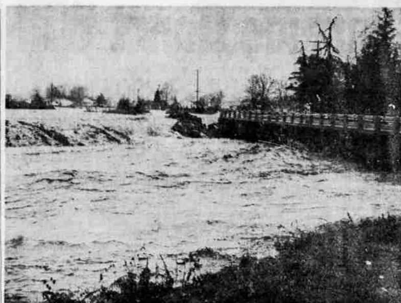
Barnett rd. bridge during flood
