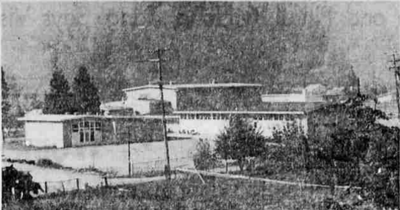
ACCEPTED BY BOARD—New additions to Happy Camp High school, seen in the foreground and at the right (with the previously existing plant in the background), recently were accepted by the Siskiyou Joint Union High School district board of trustees. The additions include classrooms which are now being occupied.
