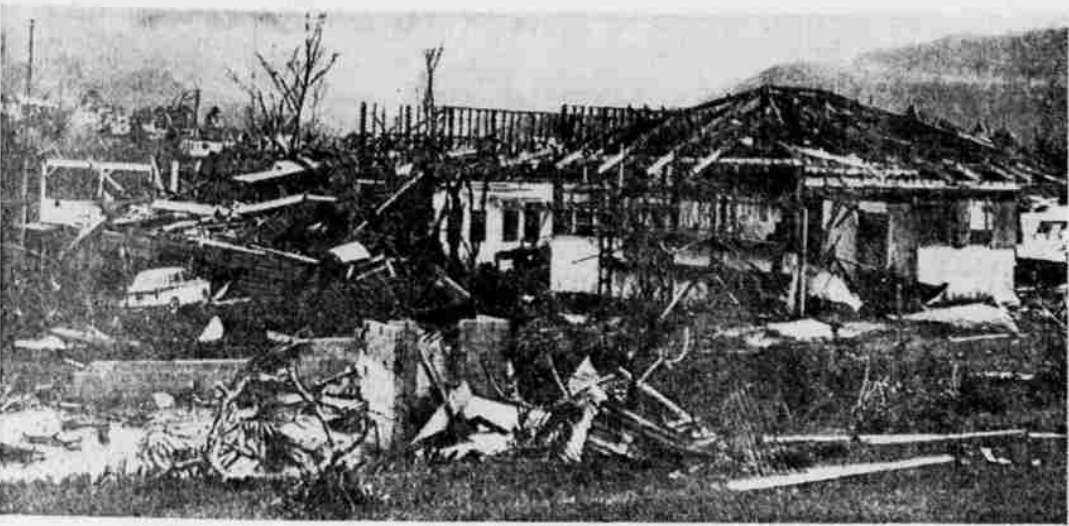
EFFECTS OF STORM —This housing project shows the effects of high winds which accompanied Typhoon Karen, devastating Guam. About 90 per cent of all housing was
