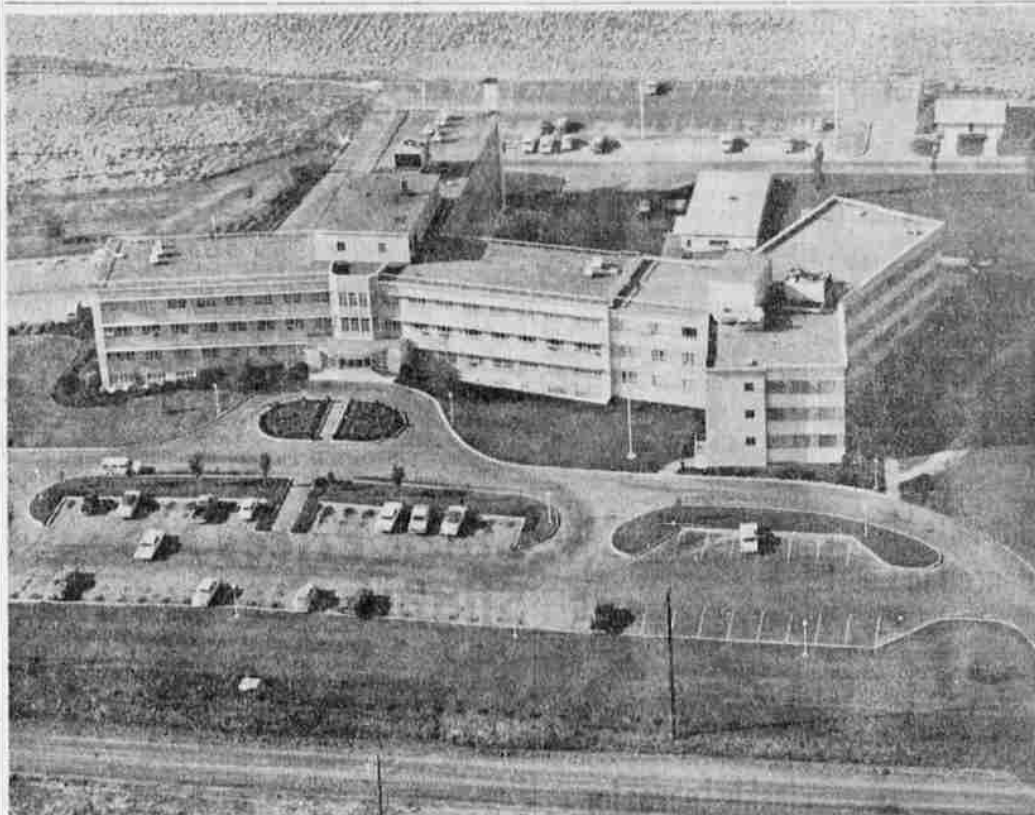
ROGUE VALLEY HOSPITAL—The annual meeting of the board of directors of Rogue Valley hospital Monday and open house Tuesday and Wednesday of the hospital's new wing will highlight activities there next week. This aerial view shows the new $2,000,000 wing (right) which was completed this fall. The 175-bed hospital includes an intensive care unit, the first of its kind in southern Oregon-northern California. The tours, open to all interested persons, will be from 2 to 4 p.m. both Nov. 20 and 21. (Knackstedt photo)
