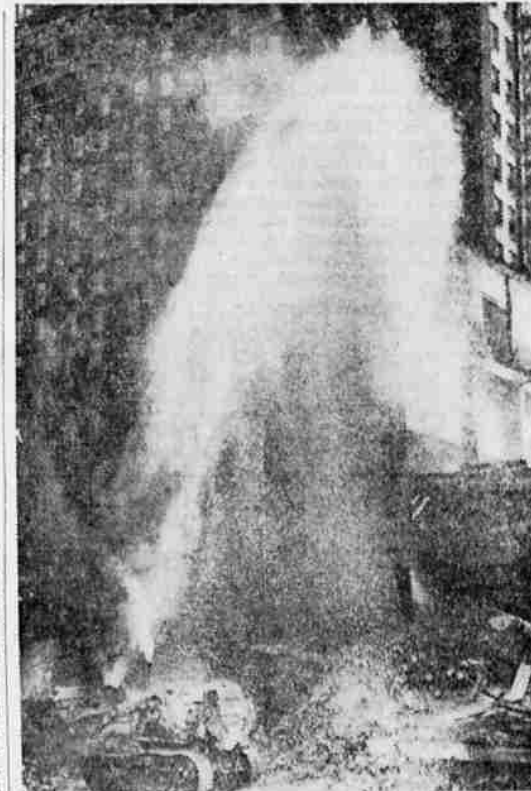
MOVES OLD BRICKS AND DEBRIS — A caterpillar moving old bricks and debris at a factory in Memphis, Tenn., Friday, which was being demolished as part of the urban renewal program, rammed into a water main, creating a downtown geyser. (UPI)
