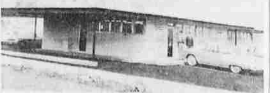
NEW HEADQUARTERS —This is the new California Highway patrol and Department of Motor Vehicles headquarters south of Yreka on old Highway 99. Standing in front of the building are Capt. C. J. McAlister and a visiting inspector, Russell Hannis.
