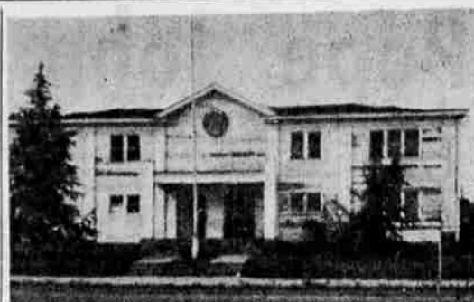
SUBJECT OF FUND DRIVE—This is the Central Point American Legion hall, erected in 1947. At present, members of the post and the community are staging a fund drive to repair and paint the building.
