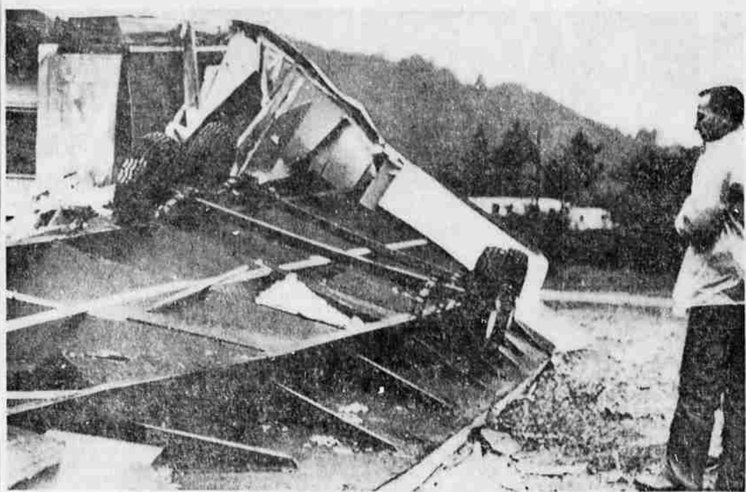
HOUSE TRAILERS DAMAGED — One of eight heavily-damaged house trailers at a Gold Beach trailer mart is shown after it was picked up by strong winds and deposited in shambles across Highway 101. (UPI)
