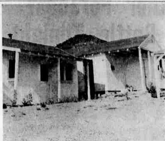
WELL-PAINTED — This group of houses helps in attracting the better pickers. Both the interior and exterior before picking season was clean and neat. Some of the cabins provided telephones.
