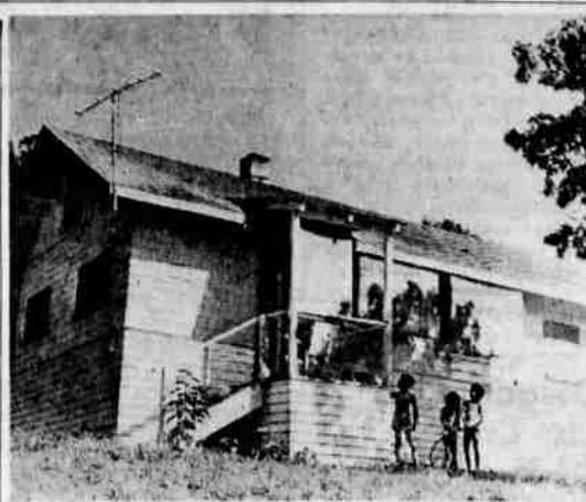
RELOCATED HOUSING — The house was moved into a local orchard before picking season started to provide comfortable quarters for a large family. More local orchardists are buying houses which for one reason or another must be moved off the original property. These provide plain, but comfortable quarters during the picking season. Note the TV antenna and bamboo blinds to keep the sun out.
