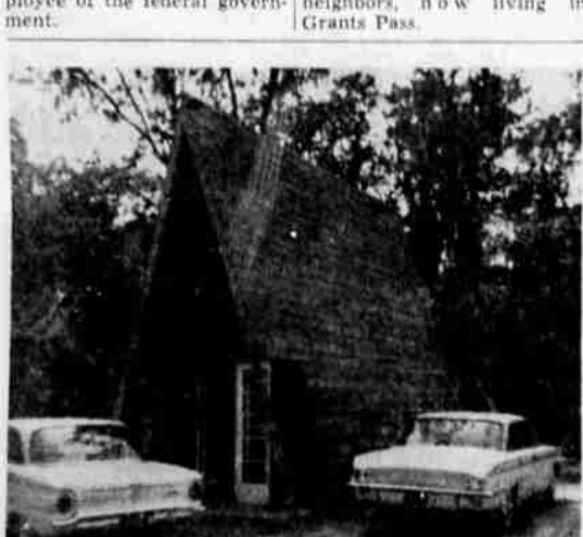
THIS IS AN OFFICE? — Yes, it really does house an office. This "A" shaped structure was built by Lloyd Whitney of 3215 Madrona L., Central Point, at a cost of some $2,000 on the Jacksonville highway near Oak Grove school.
