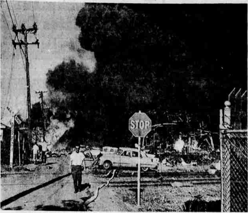
FACTORY LEVELLED — This is a general view of a fire and explosion which rocked a two-story paint factory at San Leandro, Calif., Wednesday. Fire units from nearby Oakland and Hayward were sent to battle the blaze which injured at least a dozen persons. Shock waves from the explosion blew out windows in nearby homes. (UPI)
