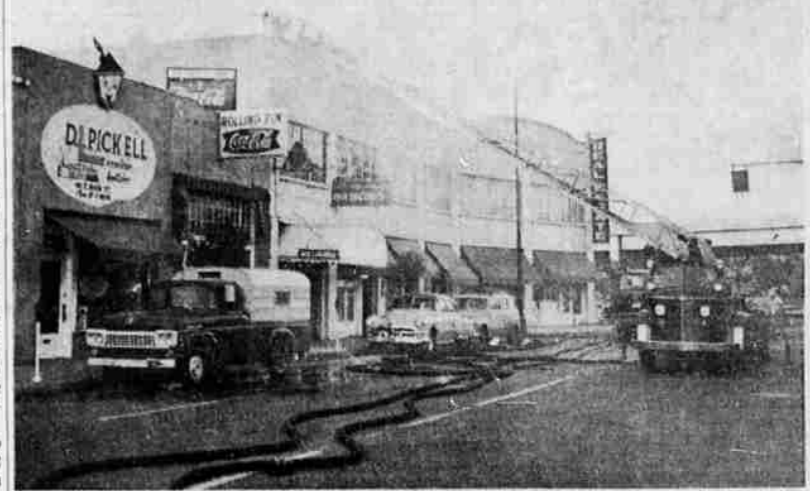
APARTMENT DAMAGED - Smoke arises from the Walker building, 419 1/2 East Main st., where an apartment was damaged by fire yesterday evening. Firemen said that the blaze occurred when a gasoline can
